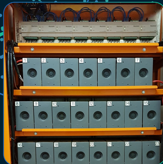
Above: BMU2408 x7 Channel installation
