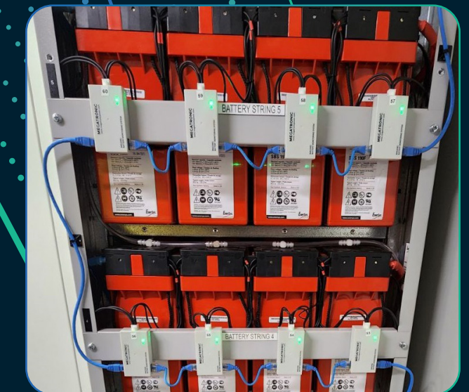
Above : BMU2401 Single Channel installation
