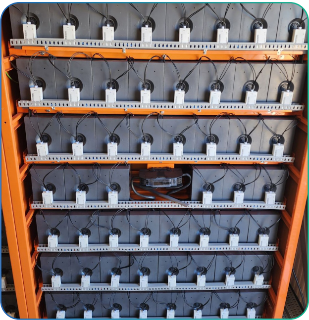
Above: BMU2401 Single Channel installation
