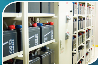
Switchroom Control Power Backup System's
